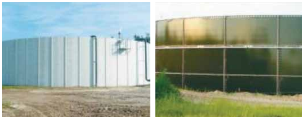
Figure 10.13 Concrete and steel tanks for liquid manure
